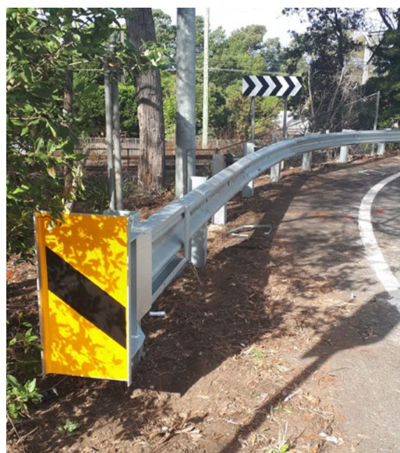
Guardrail replacement
