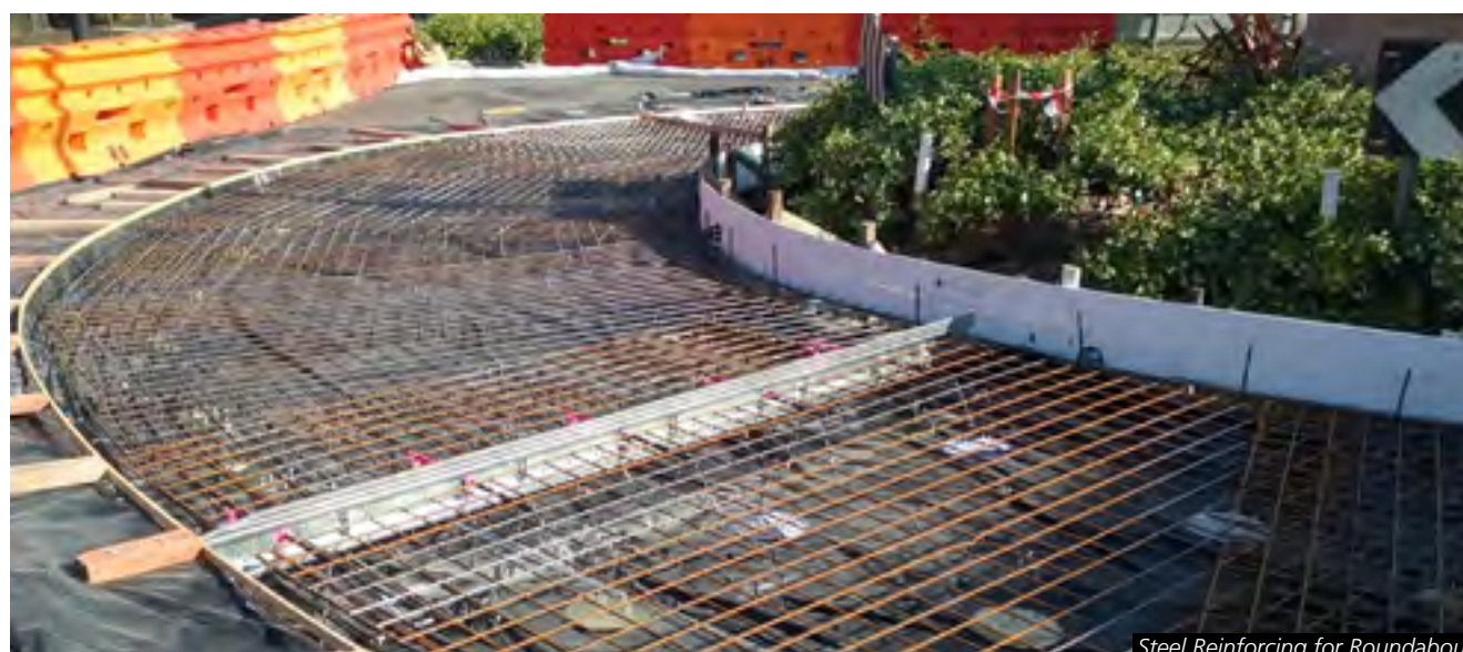
Steel Reinforcing for Roundabout
