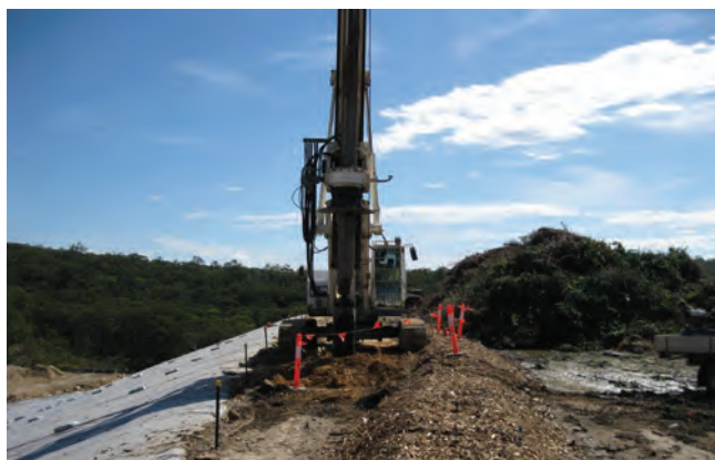
Blaxland landfill gas capture wells drilling
